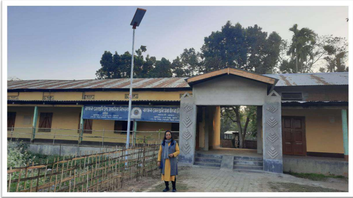
Photographs of Solar Street Light at Bangfor Village under “AAGY”
